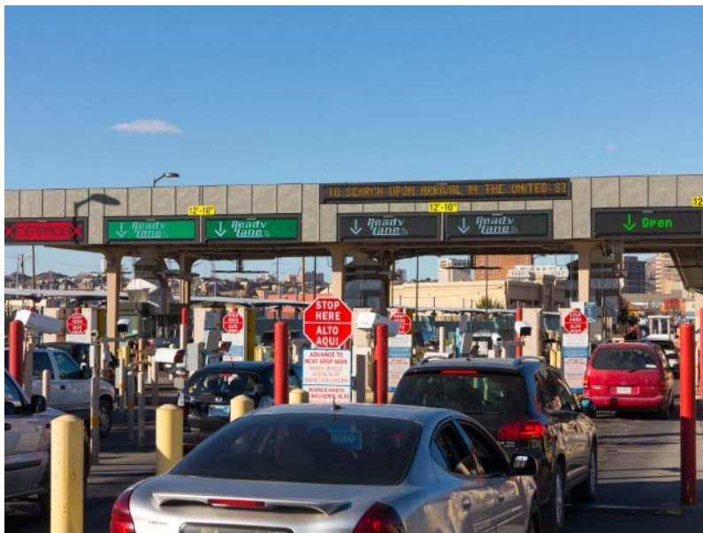
Figure D-4. Lane Management with Dynamic Signs at a CBP Primary Inspection Facility (Source: CBP).
