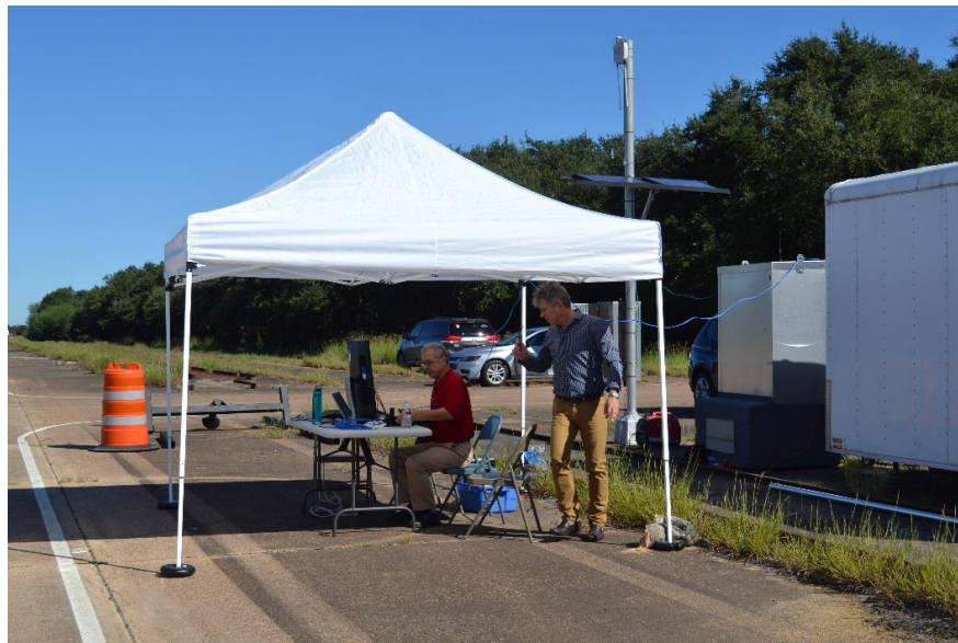
Figure 14. RSU Installed on Top of a Pole.
