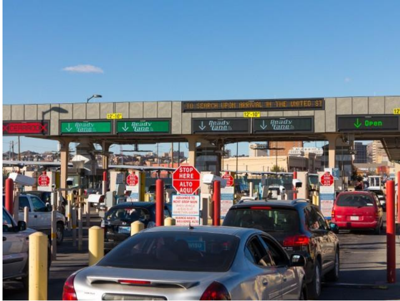
Figure 6. Lane Management with Dynamic Signs at a CBP Primary Inspection Facility (Source: CBP).
